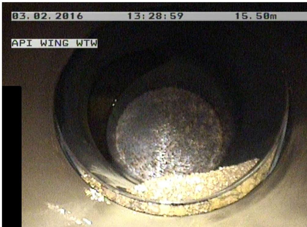
**Leak identified on wide open joint section with debris ingress identified**
