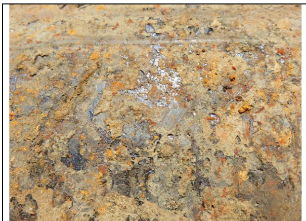
Pipe wall image
