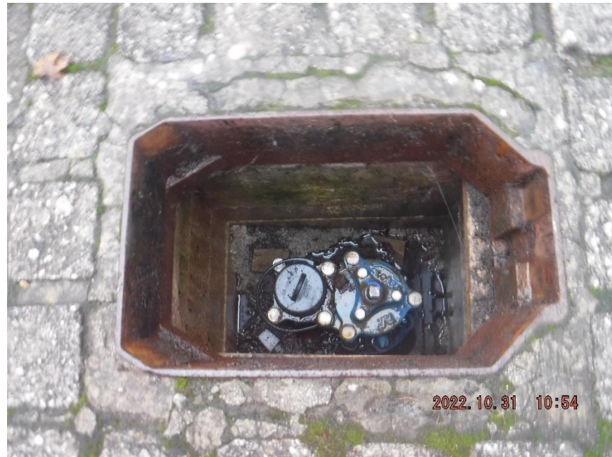
Image of hydrant cap in situ
