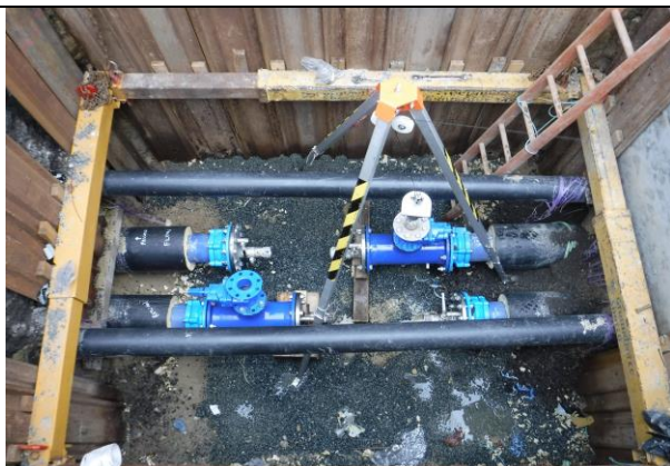
Site Location: Pipepod retrieval point
