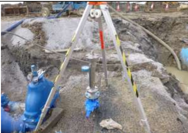
Site Location B: System entry point
