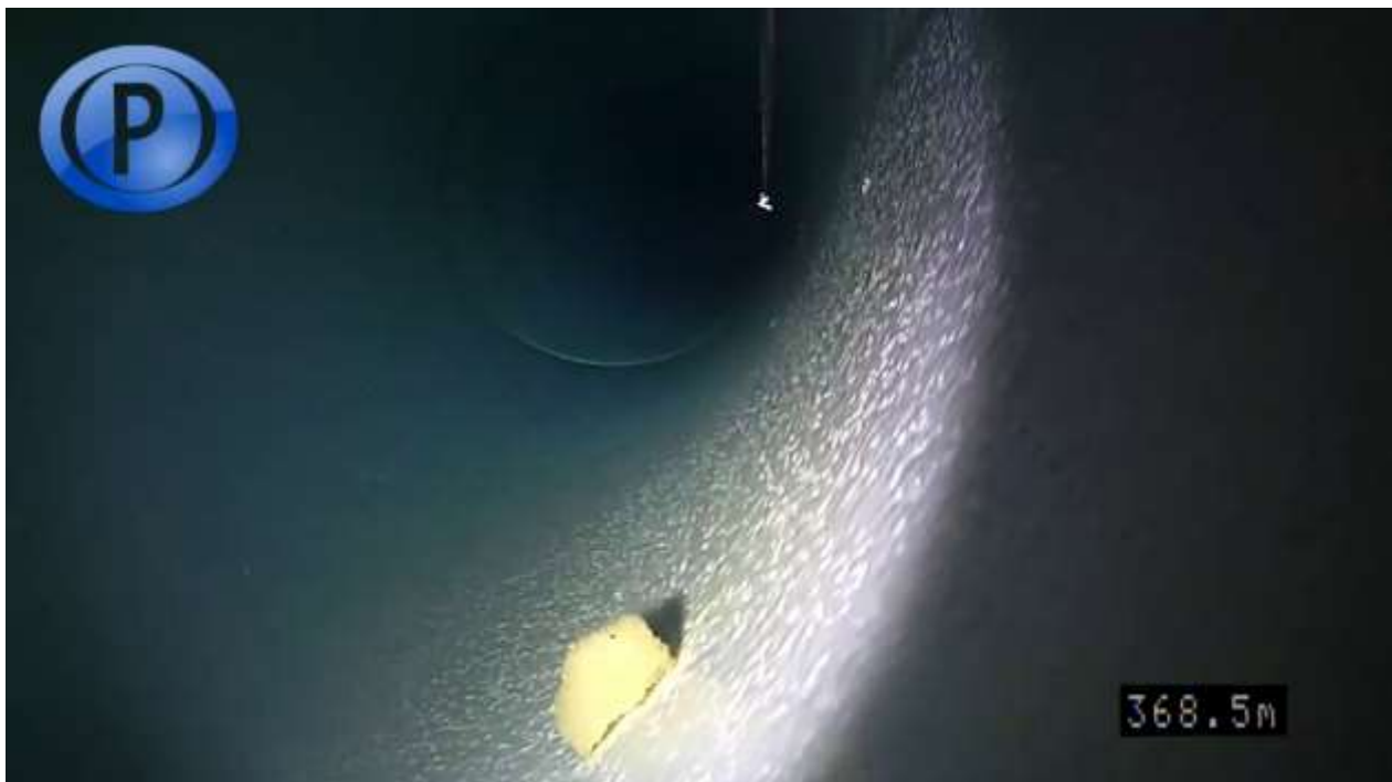
Joint image with debris identified
