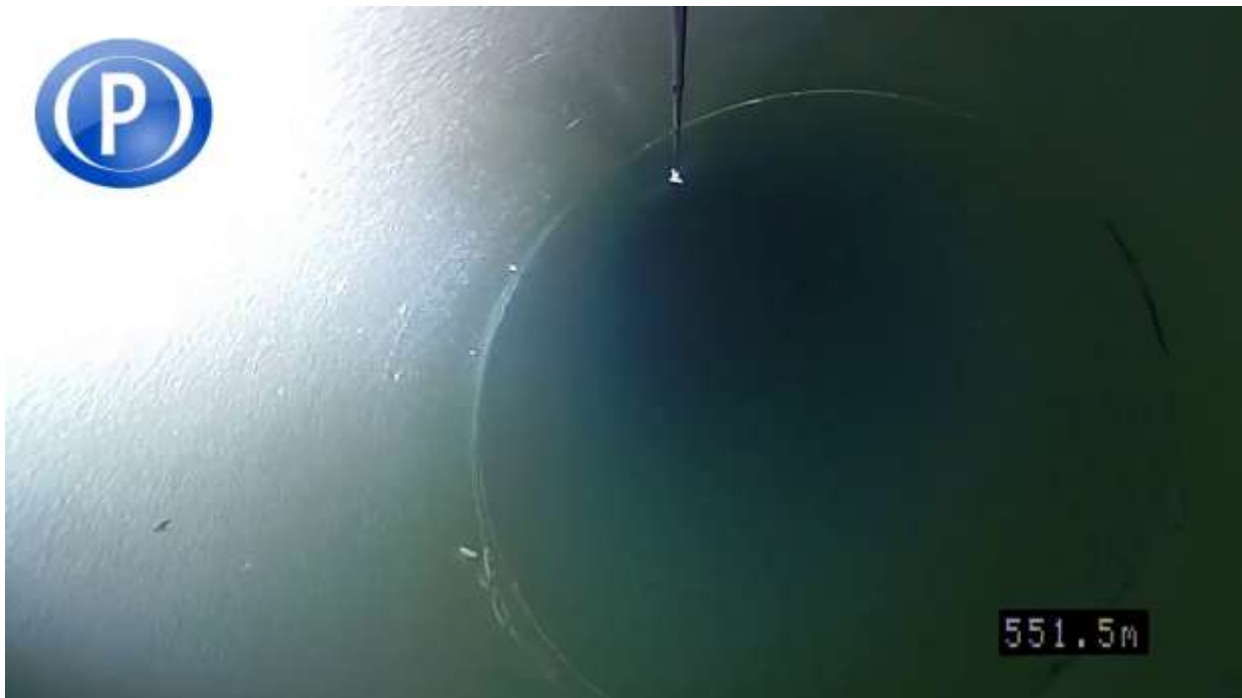
Joint image with possible gasket identified
