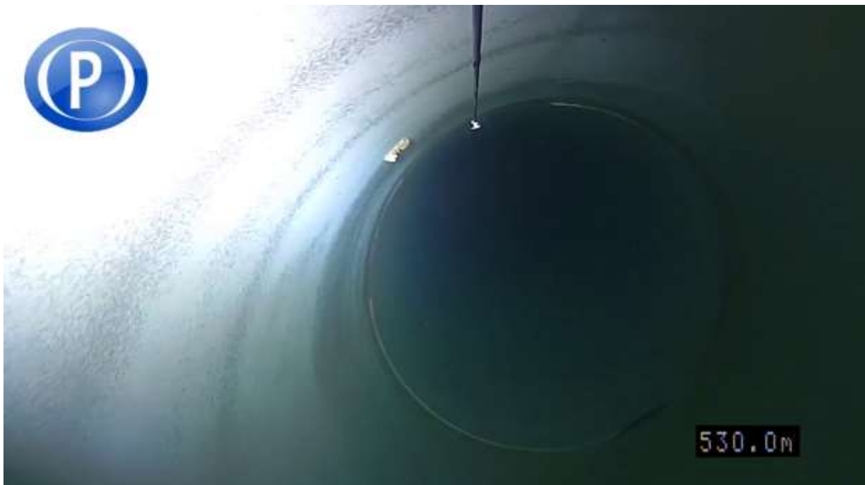
Joint image possible gasket identified
