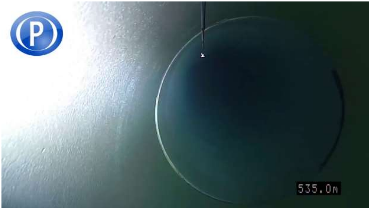
Joint image with possible gasket identified
