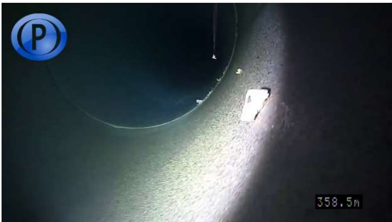
Joint image with debris identified
