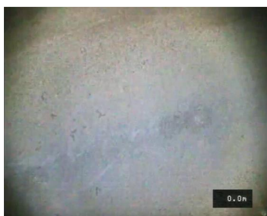
Image at pipe insertion point
