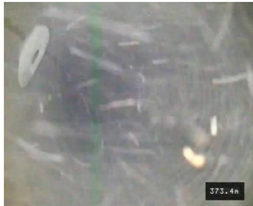
Drilled cement lining coupon identified
